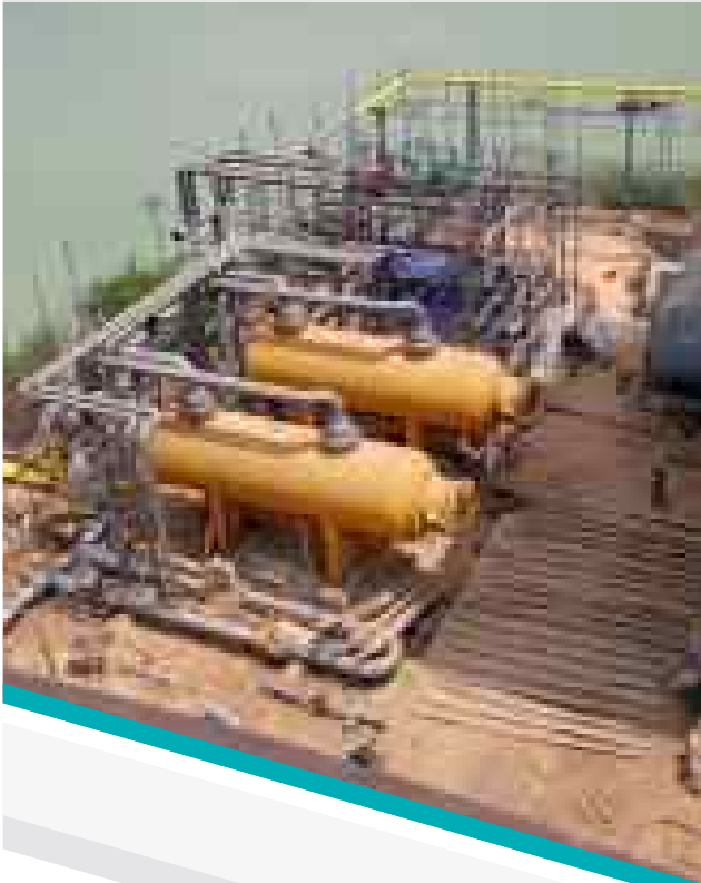
Piping Fabrication/Installation, Gas Heater, Scrubber, Valves Installation
